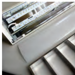
New diffuser and louvre
